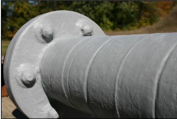
SCC Wax Wrap 80A can be applied over flanges and bolts
